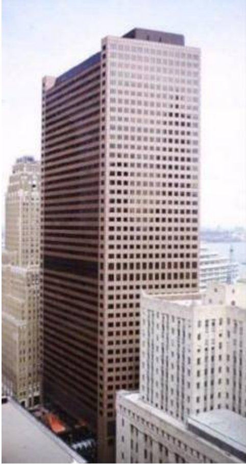
WTC 7: 47 - Story, steel-frame building..
