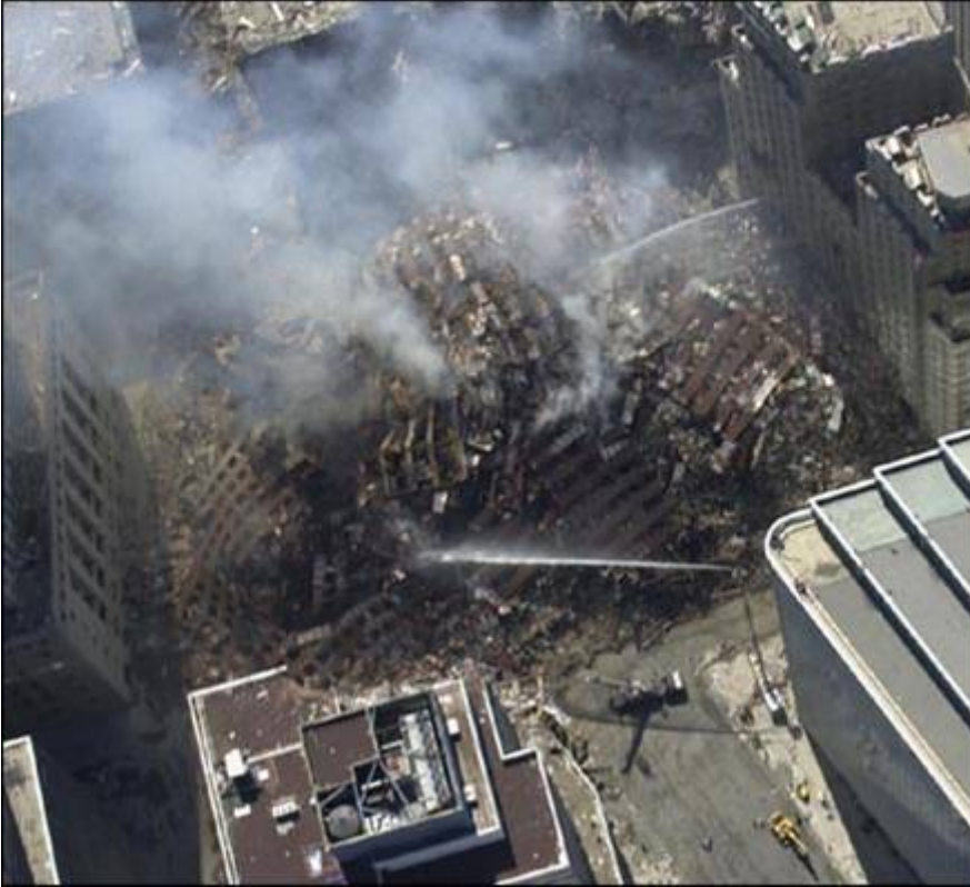
WTC 7 collapsed completely, onto its own footprint
