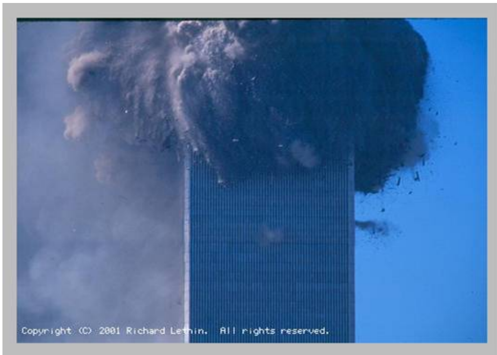
North Tower during top-down collapse.
